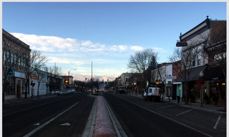
Above: Before the project, Main Street was a busy four-lane road. Below: After renovations, Main Street became friendlier to pedestrians and safer for everyone.
